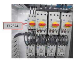
Figure 1: TD Lube Pump Motor Circuit Breaker
